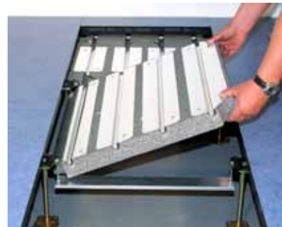
3. Installation of the heating units with heating transmission sheets.
