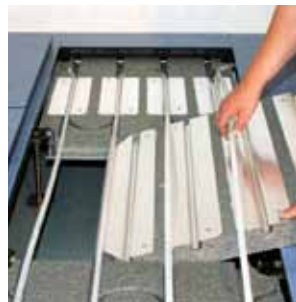
2. Unclip the heating tubes and simply remove insulating thermal unit diagonally upward. Electrical cables are now accessible.
