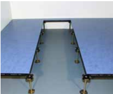
1. Lifting of panel rows for the installation of the floor heating.
