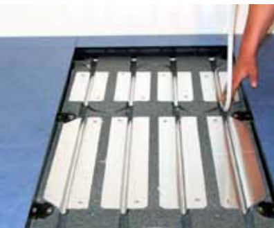
4. Installation of the heating tubes.
