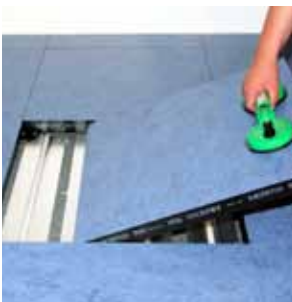
1. Panel lifting by means of uni-laterally set lifting device.
