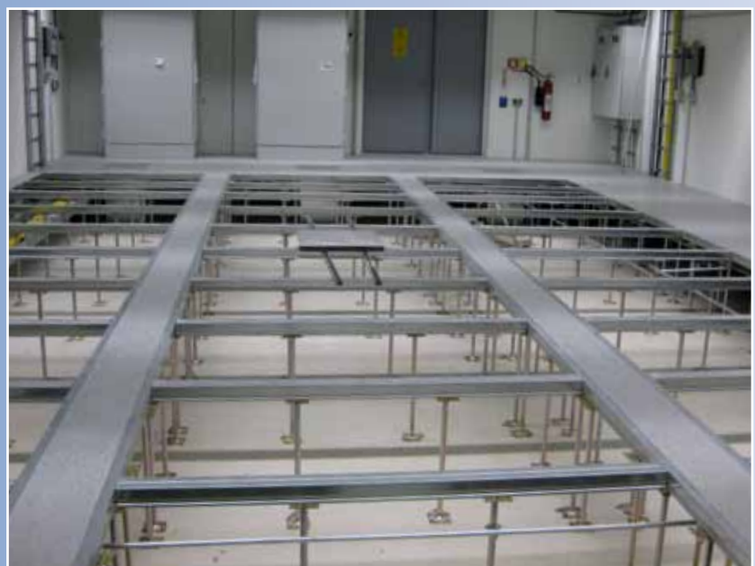
Walking area with open frames for the installation of robots
